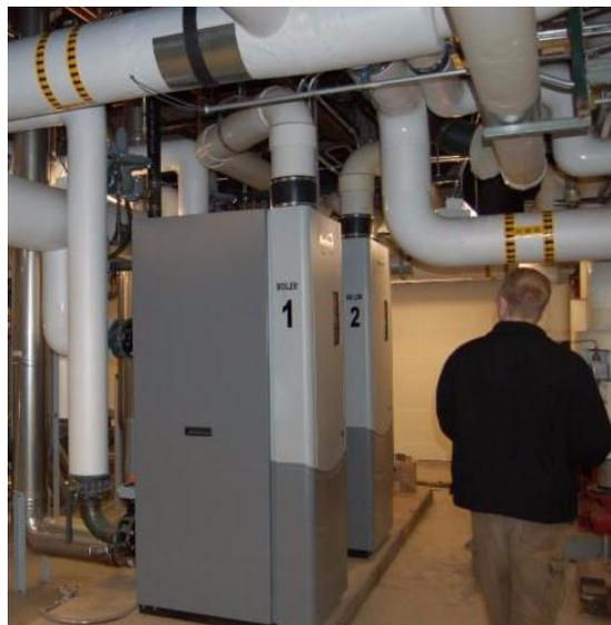
If you decide to replace your old boiler, SEDAC recommends purchasing a **high-efficiency condensing boiler that modulates**. Read more about high-efficiency condensing boilers, modulating boilers, boiler maintenance, and boiler retrofits in our [Boiler Tech Note](#).
