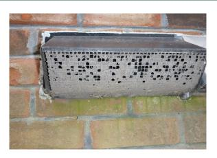
between the two, but occasional maintenance would help, too. Since the dryer cannot exhaust properly, drying uniforms takes much longer, places a far greater strain on the machine, reduces the lifespan of the drier, uses more electricity, and costs more money to run.
