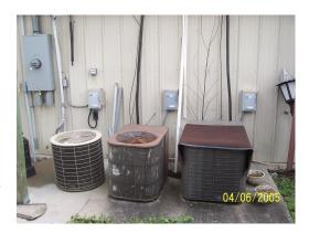
During operation, each one of these units is trying to reject heat to the environment. This task becomes much more difficult if another compressor that is trying to do the exact same thing is sitting directly next to it. The consequence is that each compressor now has to work harder to accomplish its task and equipment life is shortened.
