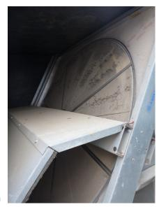
air using exhaust air and are now in many instances required by the Energy Code. These heat wheels have a lot of air that moves through them that needs to first be filtered to keep the energy wheel from getting contaminated.
