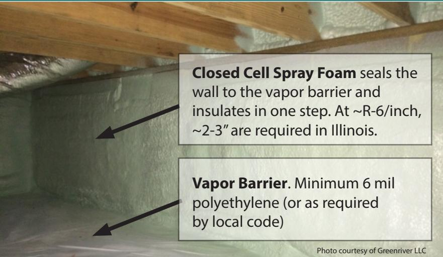
**Closed Cell Spray Foam** seals the wall to the vapor barrier and insulates in one step. At ~R-6/inch, ~2-3" are required in Illinois.
