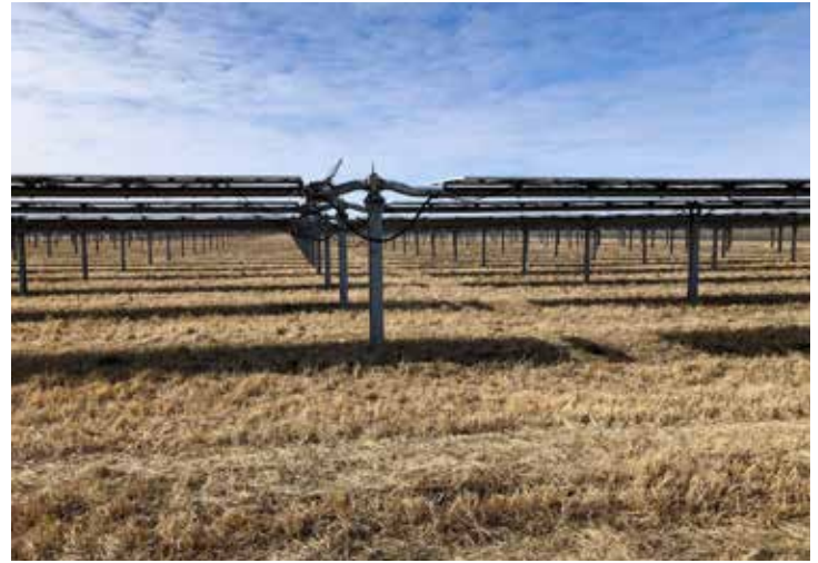
Solar array over grass
