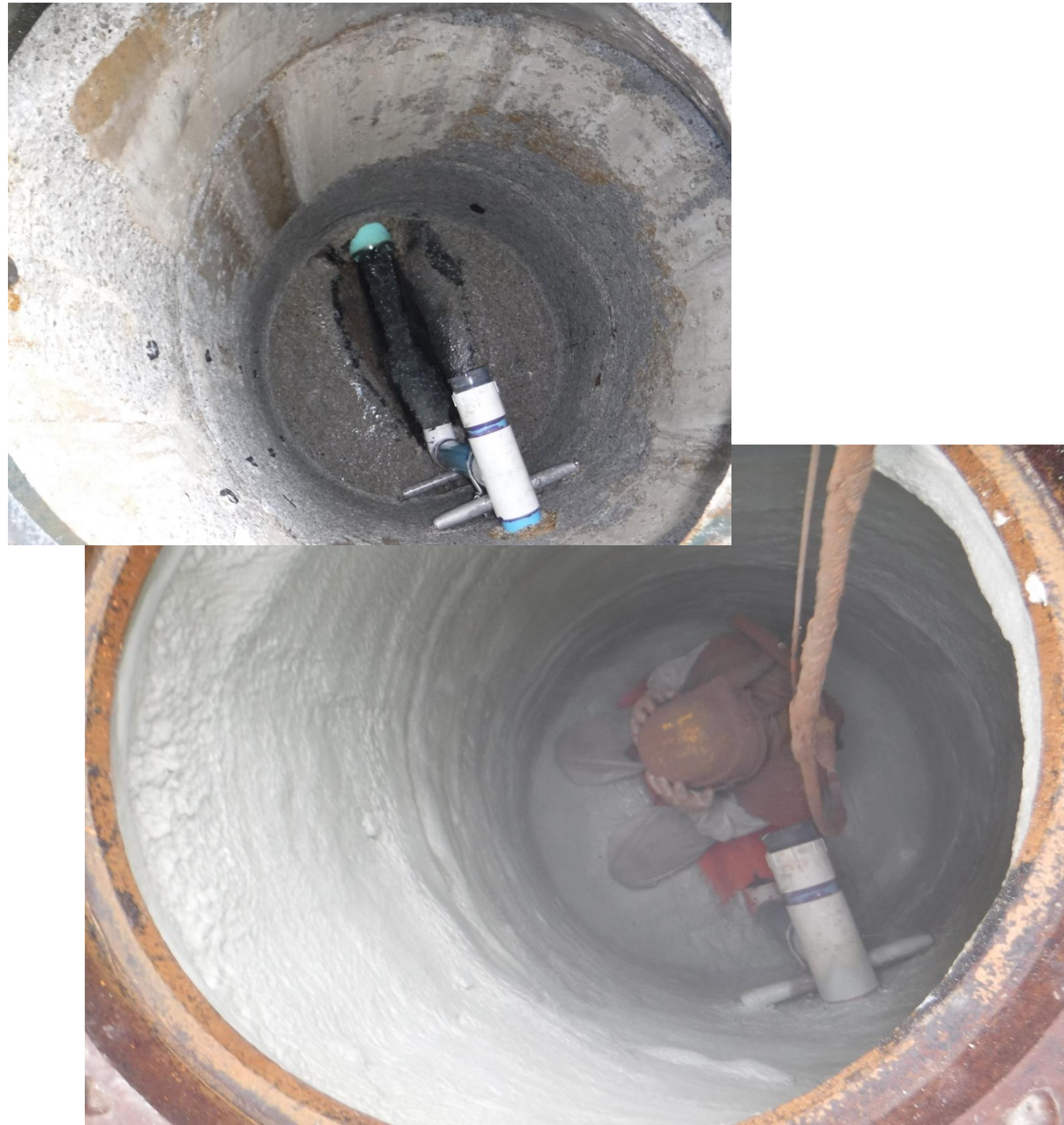
Cleaned and Prepared Manhole
