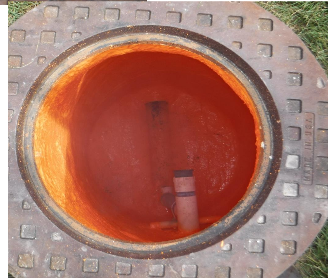
Final Barrier Layer and Completed Manhole
