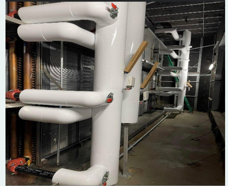
Properly insulated air- and vapor-tight system
