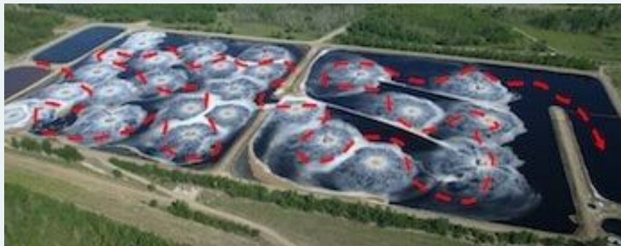
Good Flow Ensures Full Detention Time and Treatment
