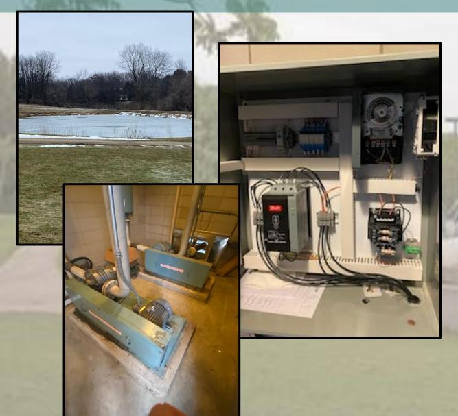
Two lagoons on site - roots blowers for aeration Smaller lagoon 2x 10HP blowers Larger lagoon 2x 20HP blowers Previously ran 24/7 Added control panel with timer controls
