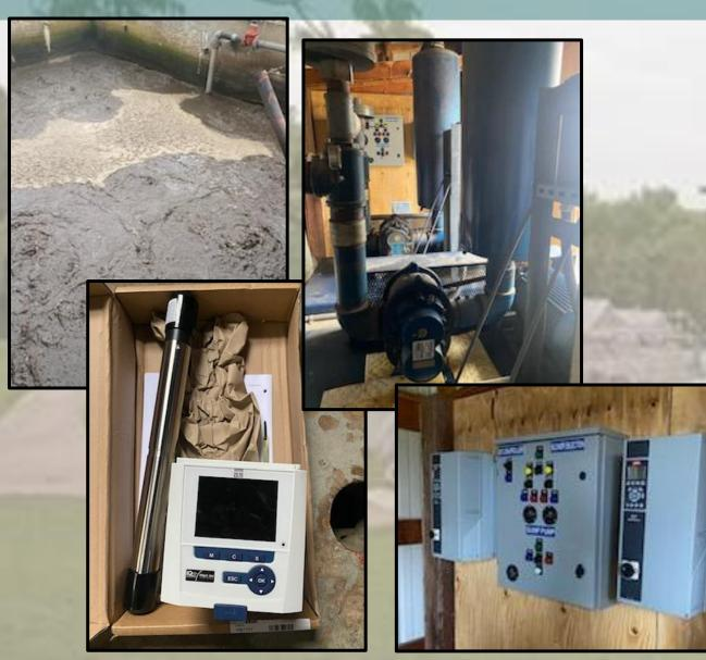
Aerobic digesters with 2x 20HP roots blowers Previously ran 24/7, on/off control Also operated an air lift for RAS Changed to include RAS pump Digesters added DO control and VFD
