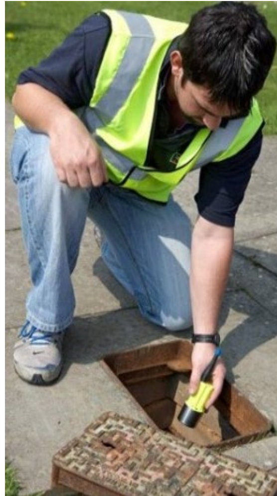
Lift-&-Shift Noise Loggers
